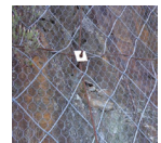
Figure 4 - Implementation of wire mesh and rock bolts on a slope composed of phyllites and metagreywackes near Coimbra (Central Portugal).
