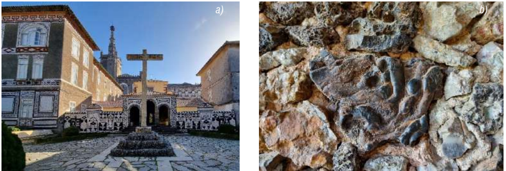
Fig 1. (a) early 17th century embrechado decoration on the western façade of the Convento de Santa Cruz do Bussaco. The dark component is provided by slag from bloomery iron smelting. (b) detail of embrechado decoration inside the entrance hall of the Convento, showing a block of tapped bloomery iron smelting slag. The chemistry of the slag is compatible with the smelting of iron ore hosted by the Ordovician Porto de Santa Ana Formation, as seen at the ancient smelting sites such as Vinha da Leira Má (Louredo) and 'Pedras Negras' (Vicariça).
